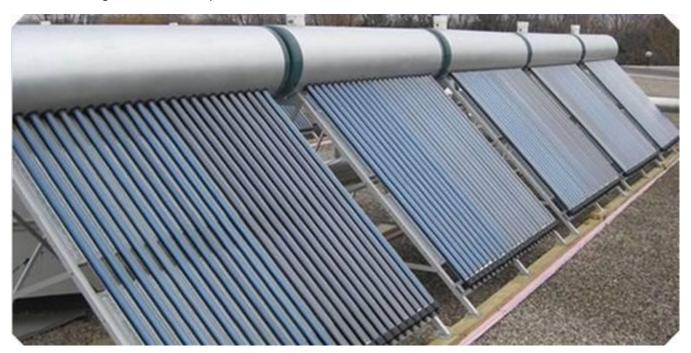
Fig. 6 Glass-Glass Evacuated Tubes Absorber
