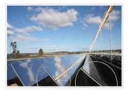
These are several mirrors which have been arranged and sharing the same receiver. Frensel reflectors have the advantage of reduced tracking mechanism complexity. They are also stationary absorbers.
